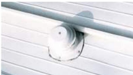
Ballew's Roof-Over System uses a specially formulated tar tape to seal vents against leaks and water damage.
